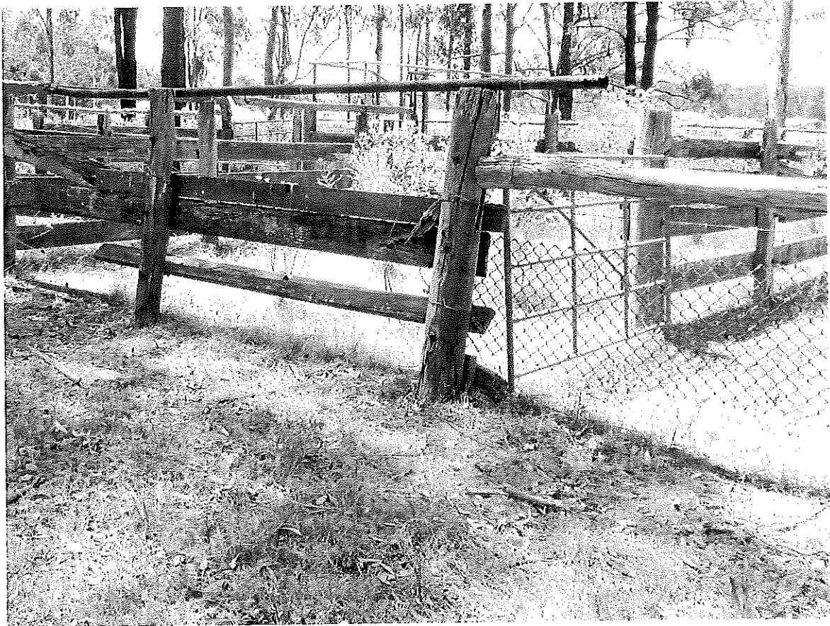
Photograph 4 – Stockyard North western Corner
