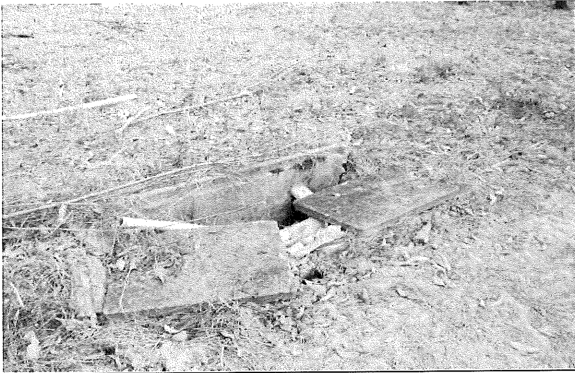
Photograph 3 – Telecommunication pit on eastern boundary of Lot 42
