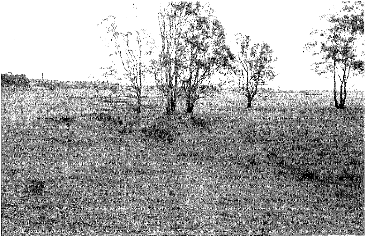
Photograph 1 – Filled areas around the western dam and gully line
